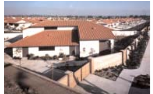
The Upland Hills Water Reclamation Plant in Upland, Calif., is an enclosed treatment facility immediately adjacent to a residential development. The plant has been in operation for almost 20 years.
